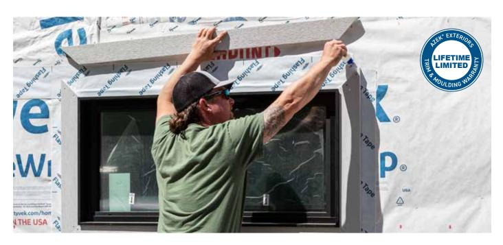
AZEK's lightweight and durable trim made from engineered polymer lasts longer than wood but can be cut, drilled, and fastened with standard woodworking tools. **See inside to learn key installation differences and best practices.**
