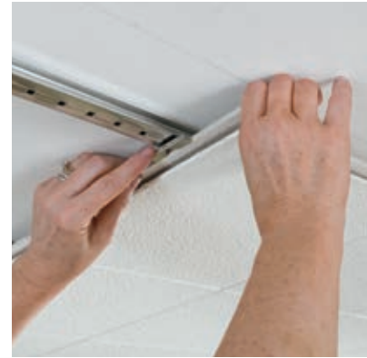
3 Position tile or plank; slide and secure clip
