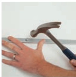
1 Install wall molding
