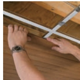
Position planks; slide and secure clips
