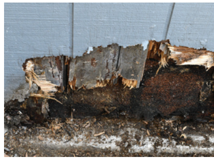
ENGINEERED WOOD Rot starts small and grows up.
