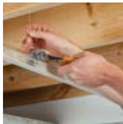
2 Suspend main beams with hanging hardware
