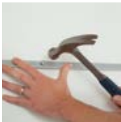
1 Install wall molding
