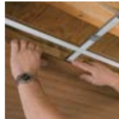
Position planks; slide and secure clips
